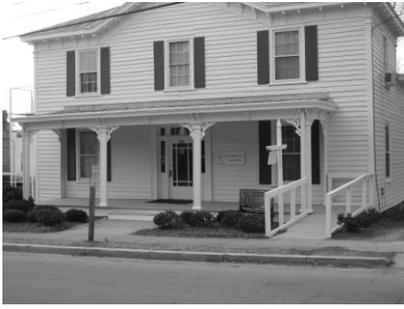
***A simply detailed wooden ramp provides access to this front porch. The placement of the ramp on the side of the minimizes its visual impact. On the opposite page, a compatible brick and concrete ramp constructed along the church's side elevation provides access to the front entrance.***
