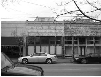
***A sound paint film must be applied to these cast iron store fronts to prevent corrosion.***
