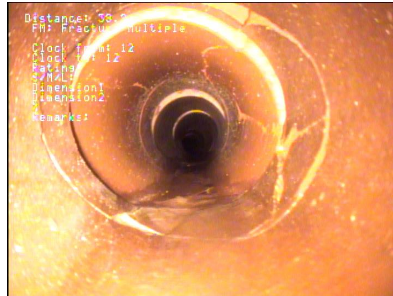
Severe Offset/Fracture
