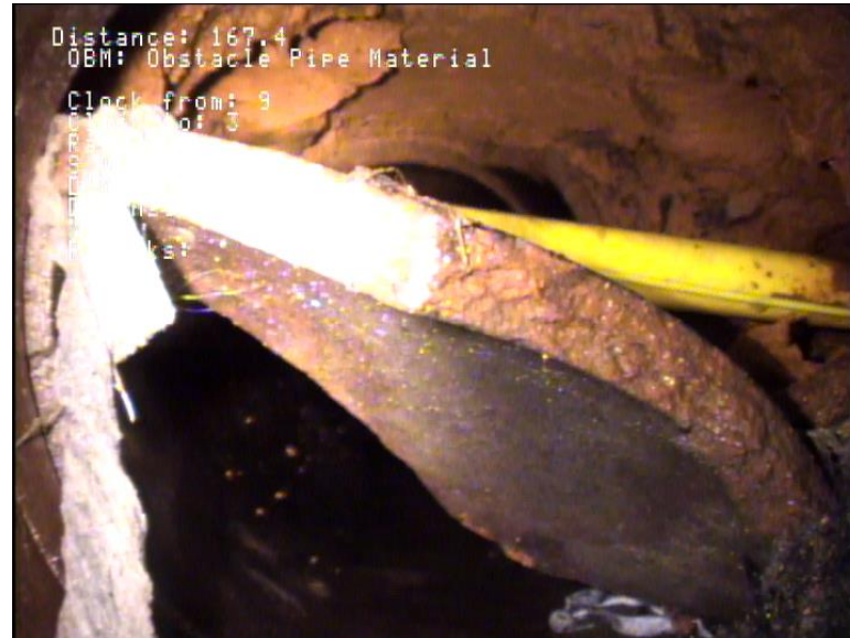
Gas Line installed through Sewer Pipe
