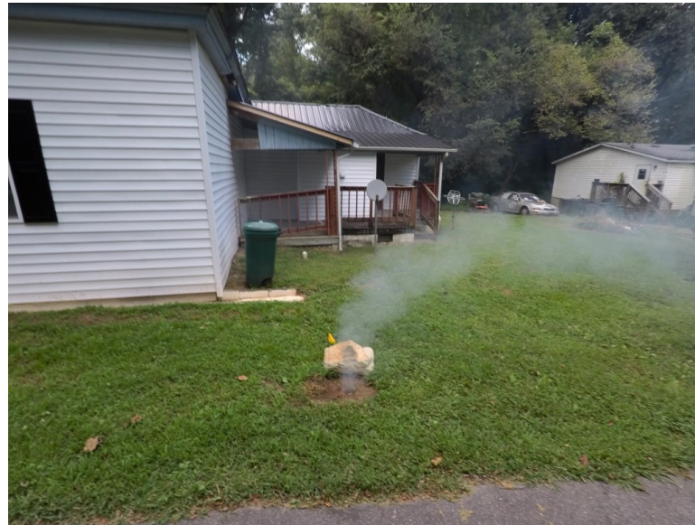
Leaking Clean-Out Cap
