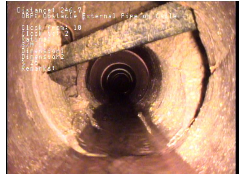
Cable installed through Sewer Pipe
