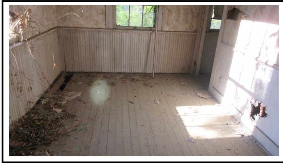
Photograph 7: A view of the wood flooring, ground floor east.
