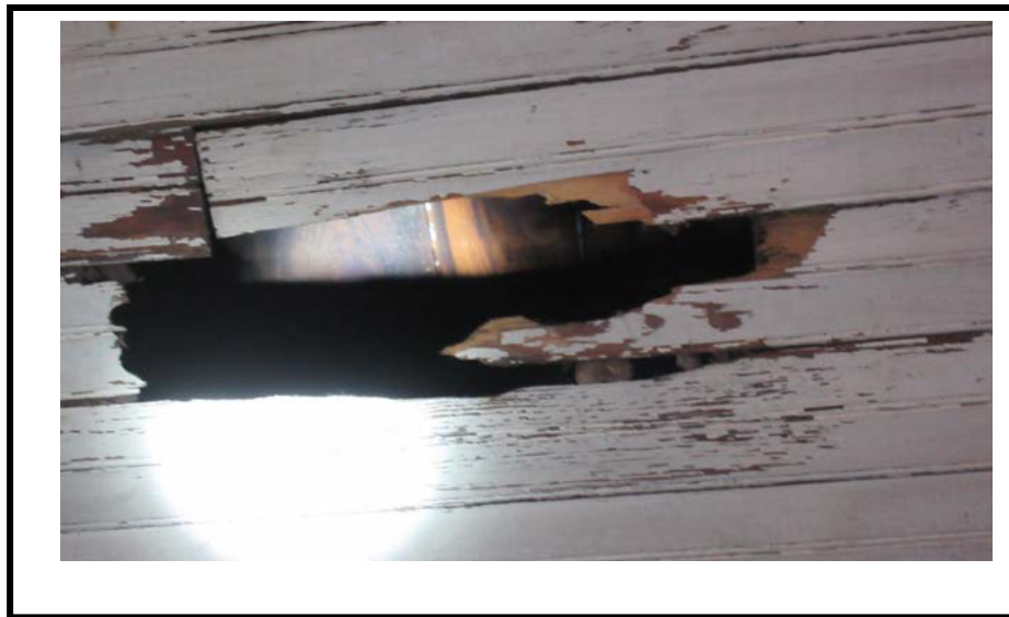
Photograph 12: A view the roof and ceiling insulation.
