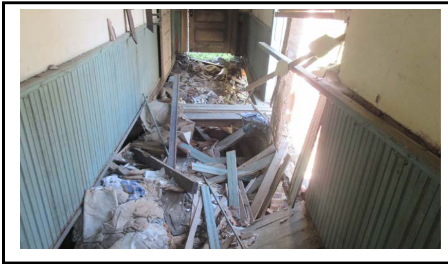
Photograph 10: A view of the collapsed floor in the hall on the ground floor north side.
