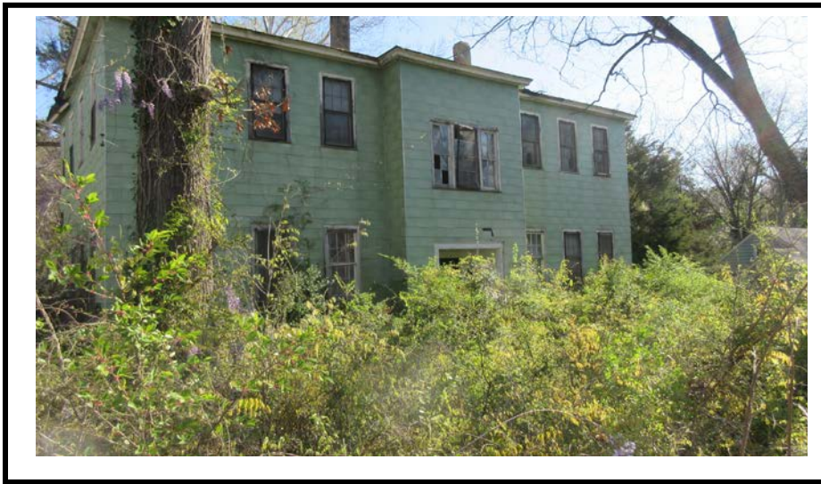
Photograph 2: A view of the building viewed to the northeast.
