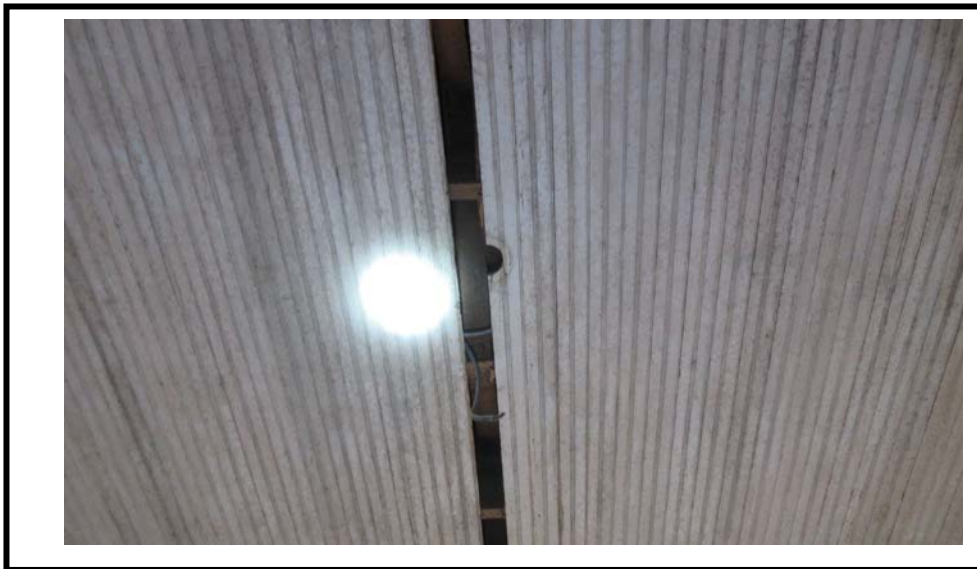
Photograph 8: A view of the wooden roof joists.
