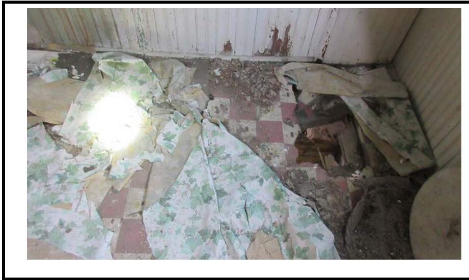
Photograph 9: A view of interior VFT flooring and partially collapsed floor in the bathroom on the ground floor east.
