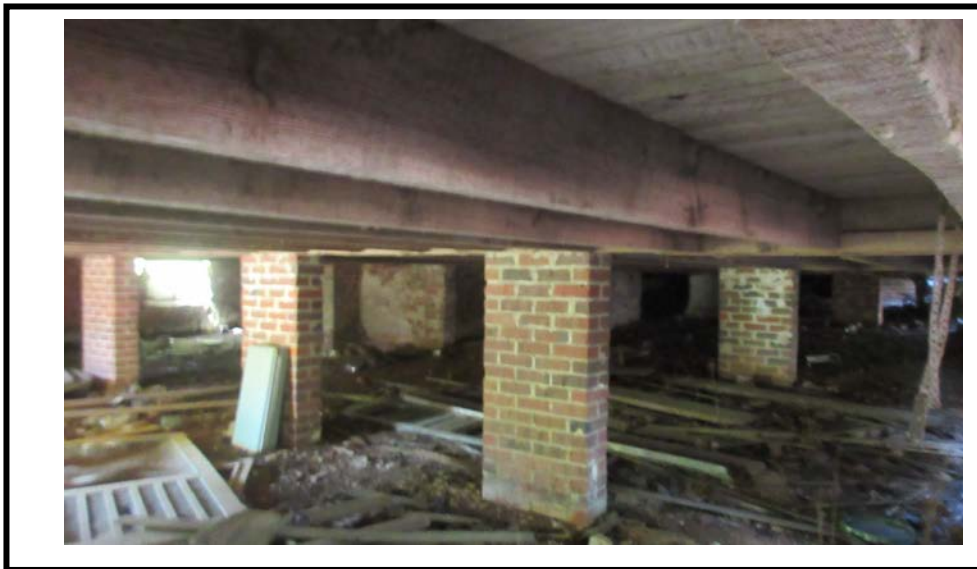
Photograph 16: A view of the crawlspace.
