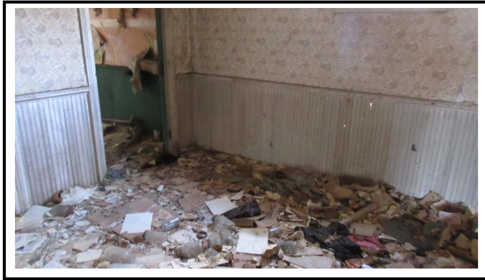
Photograph 15: A view of the second floor west.
