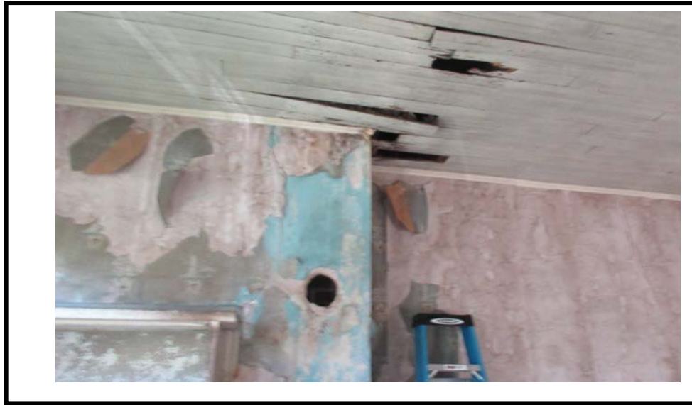
Photograph 13: A view of interior ceiling second floor east side.
