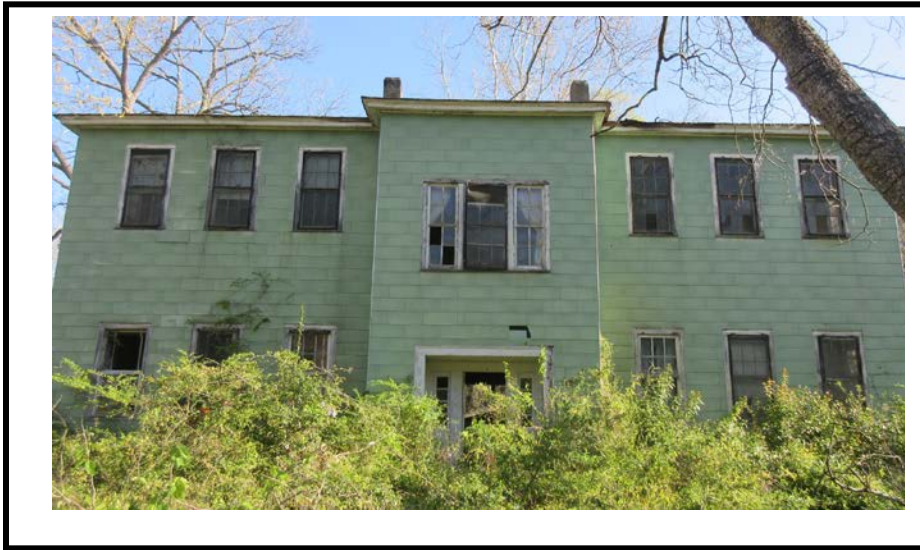
Photograph 1: A view of the building viewed to the north. Exterior green siding is transite and ACM.
